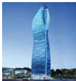
TUNED MASS DAMPERS
