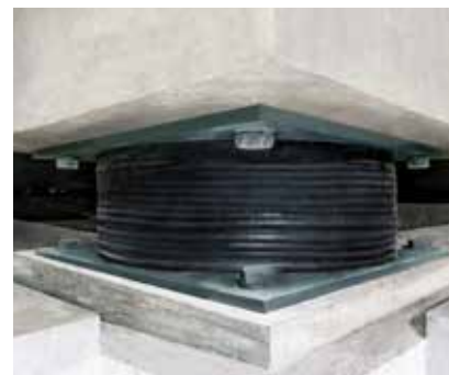
One of the 243 lead rubber bearings between the upper concrete platform and the lower concrete trough. Clearly visible are the ring-shaped deformations of the elastomer due to elastomer-steel plate layering.
