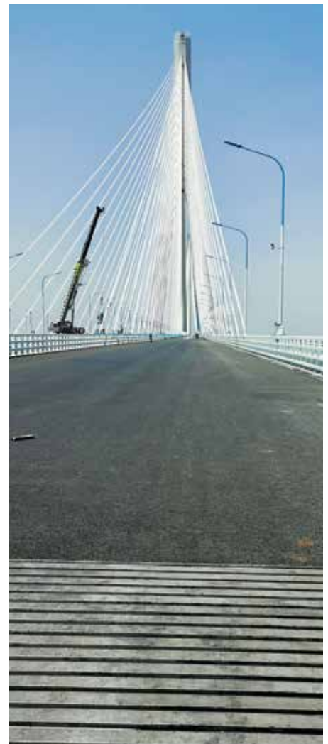
Record bridge in China: the Hutong bridge featuring a length of 11 km with the central cable-stayed bridge with a length of 1,092 m
